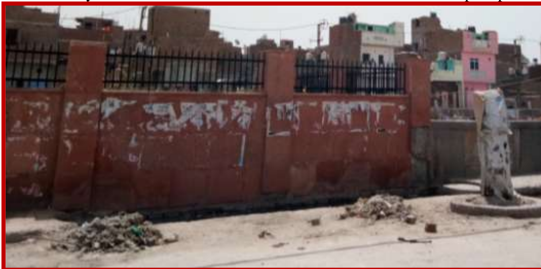
Figure 1 – Bad conditions of drains and solid waste not collected by Municipal corporations
